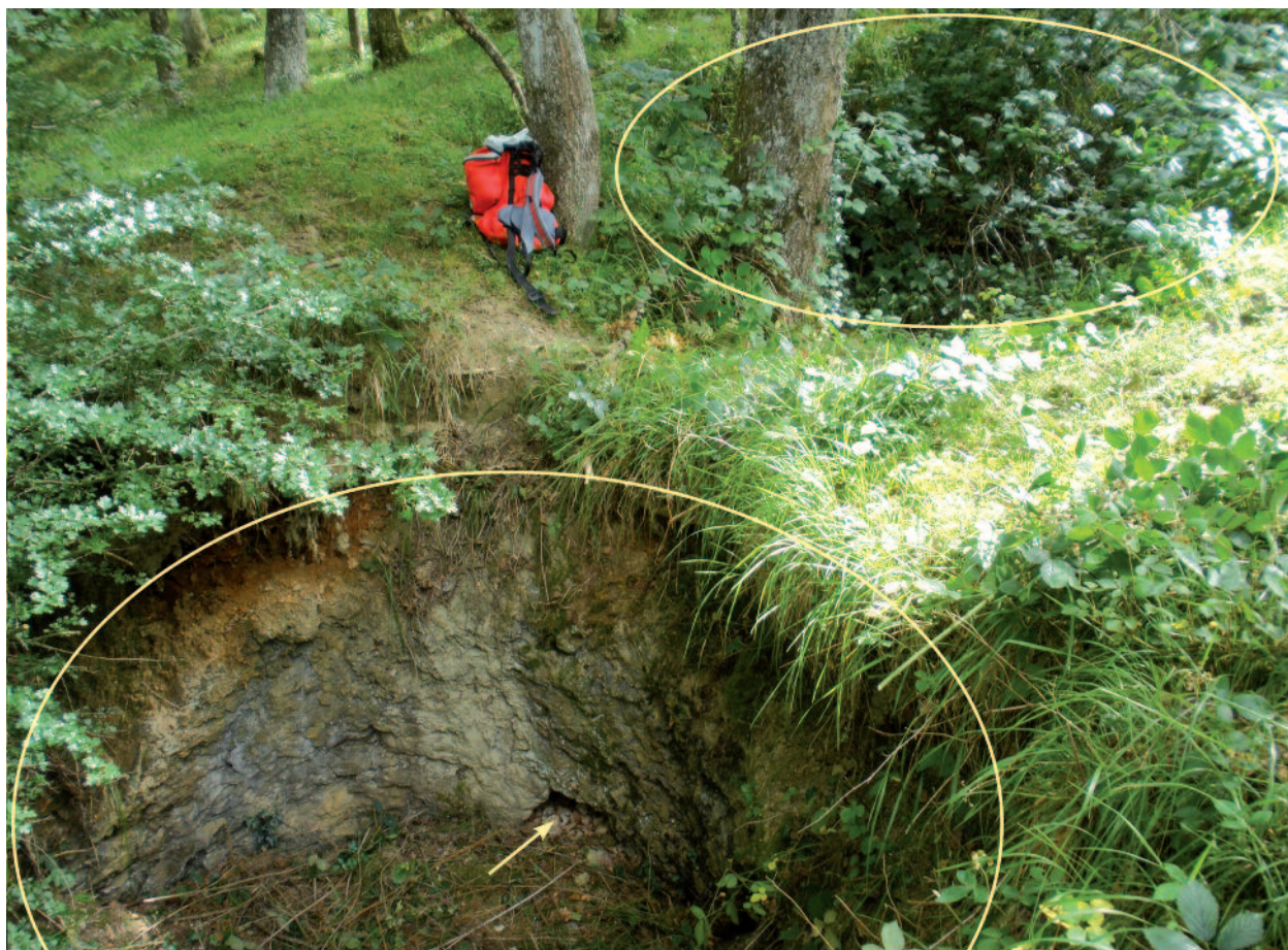
Figure 10. Double furnace of Amezola (Aramaio), where the presence of two shafts separated by a 1 m wall can be noticed. The arrow points to the opening connecting the two.
